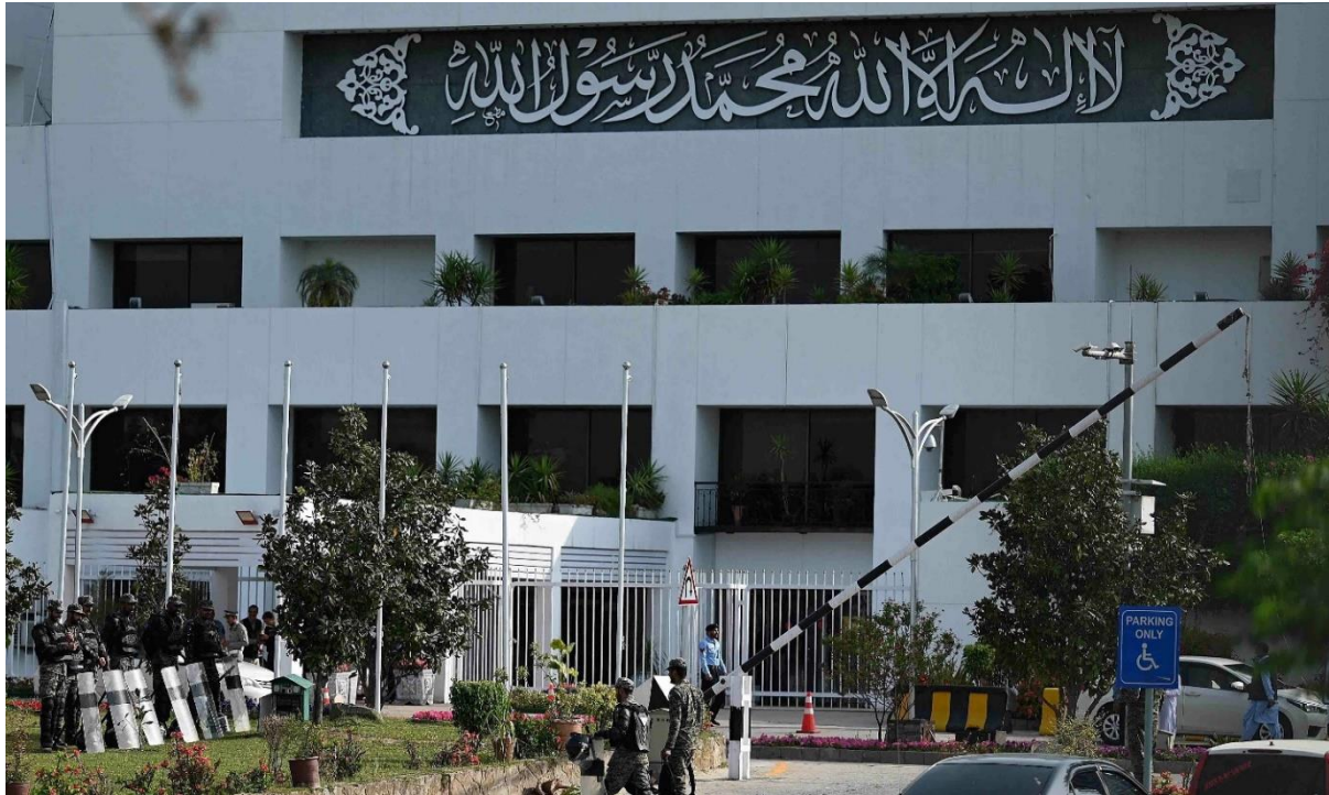
Security Personnel deployed in front Parliament House Building in Islamabad, April 3, 2022.
