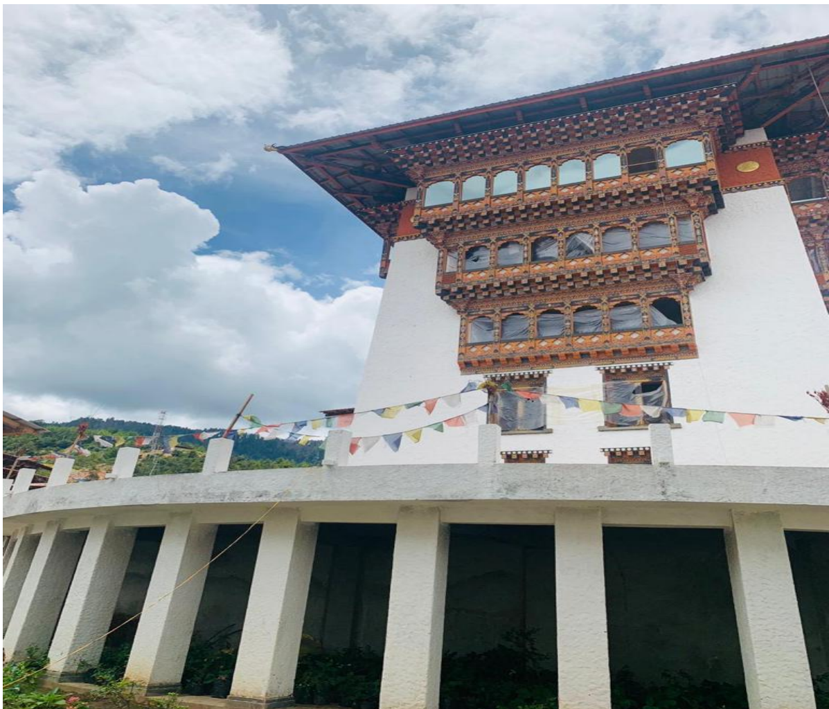
The under-construction law school in Paro, Bhutan. Source: Twitter/@DDIndialive
