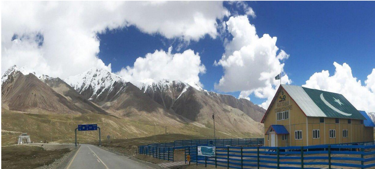
Optical fibre cables laid under CPEC projects have been operationalised from Khunjrab to Islamabad. A data centre, July 12, 2020. Source: Twitter/@AsimSBajwa
