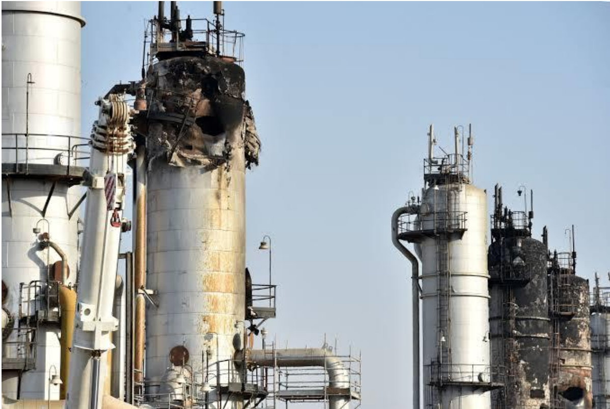
Damage to Saudi oil facilities due to the missile attack claimed by the Houthis rebels, September 14, 2019 Source: Evening Standard
