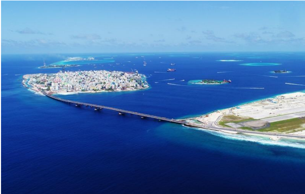
This aerial view shows the China-Maldives Friendship Bridge, which joins the capital city of Male with the airport island, Hulhule. Source: China Daily
