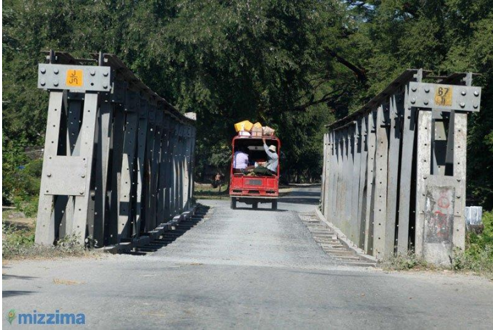
This photograph shows the Myanmar-India trade route near Tamu - a border town. Road transportation between India and Myanmar got a boost when the Indian cabinet approved in December 2015, the construction of 69 bridges including approach roads on the Tamu-Kyigone-Kalewa (TKK) road section of the trilateral highway in Myanmar. Source: Hong Sar/Mizzima
