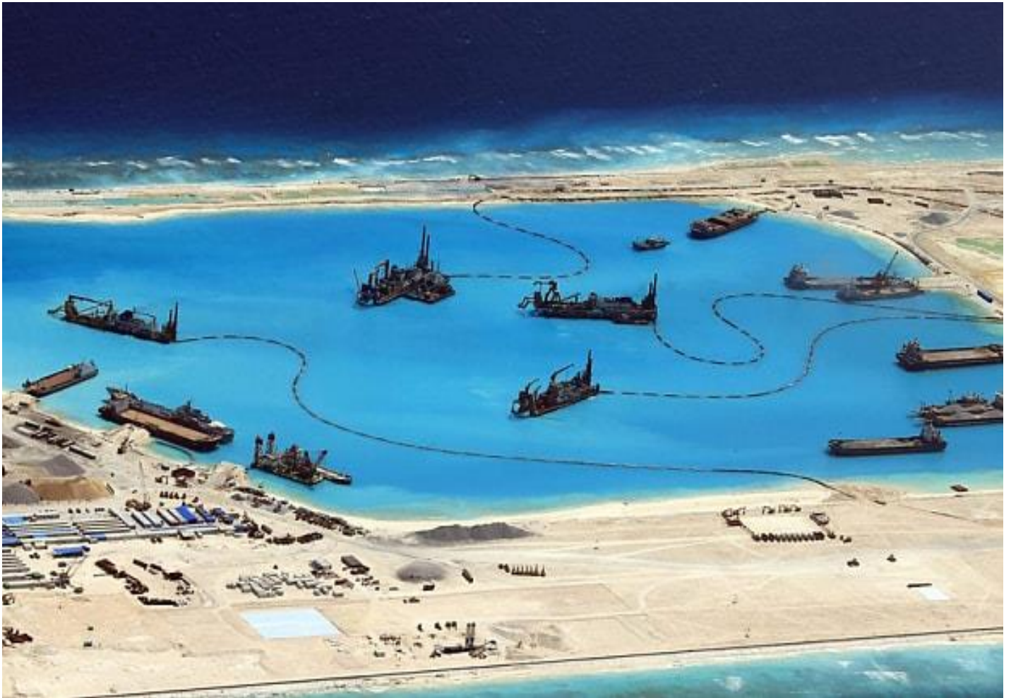
Construction by China at Kagitingan (Fiery Cross) Reef in the disputed Spratly Islands in the South China Sea. Source: EPA
