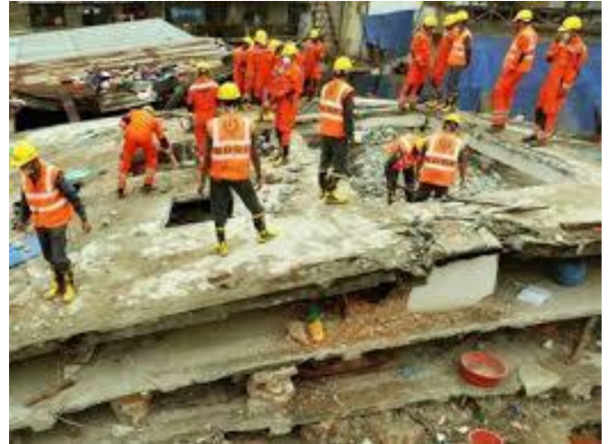
NDRF personnel conducting collapsed structure rescue operations.
