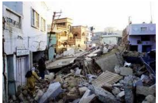
Damage to urban areas - the Bhuj Earthquake 2001. (Source: USGS)
